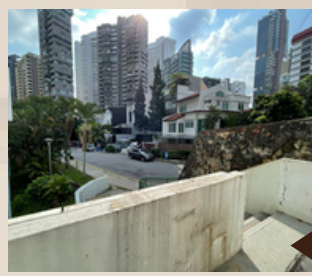
C3 & C4 Exit: Level 3 Exit to Jalan Elok
