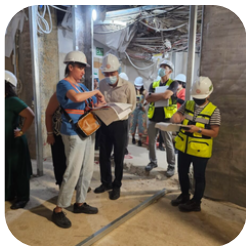
Dr Ong's Site Visit during Construction
