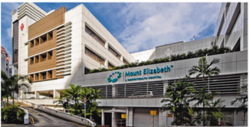
The renovation at Mount Elizabeth Hospital will take place in phases so that major clinical services can continue. A wall-breaking ceremony was held on Tuesday. PHOTO PARKWAY LIFE REIT
