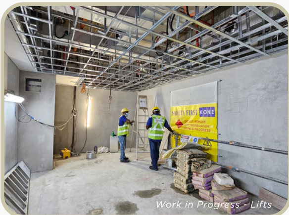
New Smoke Stop Lobby
